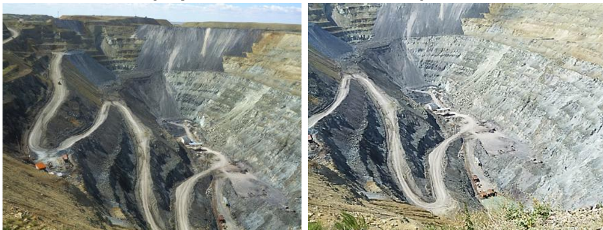
Figure 4. A large quarry near the city of Khromtau
